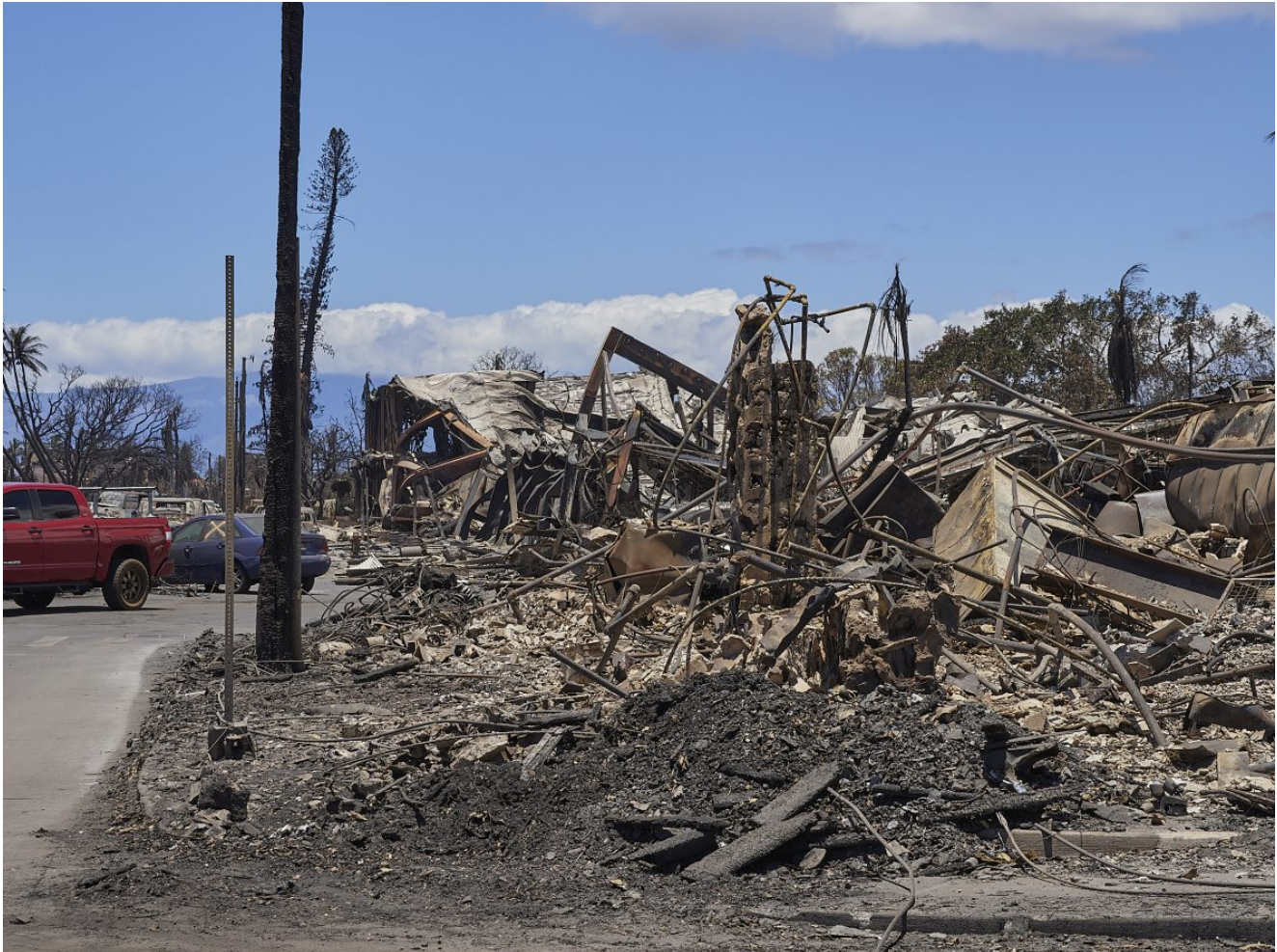
Burned stores reveal the ferocity of the Aug. 8 fire that stormed through Lahaina leaving little to nothing left at every place it touched. (David Croxford/Civil Beat/2023)
